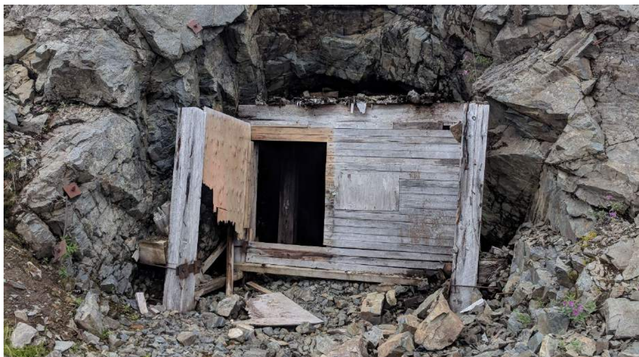
Photo 5: Portal of Doc Property adit accessing the Q17 vein
